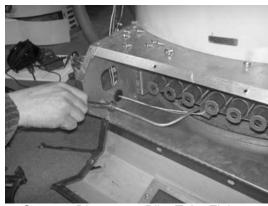
Step 10: Disconnect Pilot Tube Fitting from inside Burner Box
